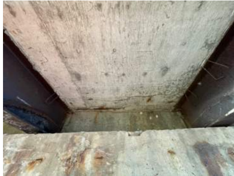
Deck Soffit - Interior - SU2 between G4/G5. Note: Typical spalls with exposed rebar, delamination and rust
