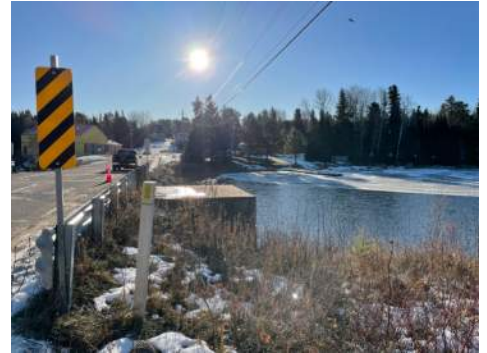
Upstream looking West
