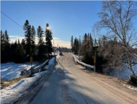
Roadway looking West
