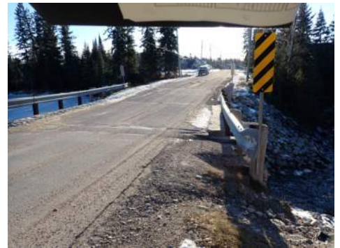
North railing - Looking West
