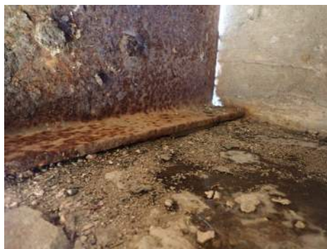
Typical exterior bearing - SU2.
