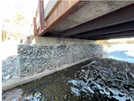
SU1 East abutment
