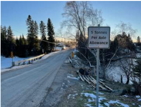
Typical Sign - NE.
