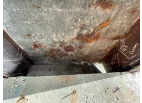
Deck Soffit - Interior - SU1 between G1/G2. Note: Spall with temporary repair, and delamination.
