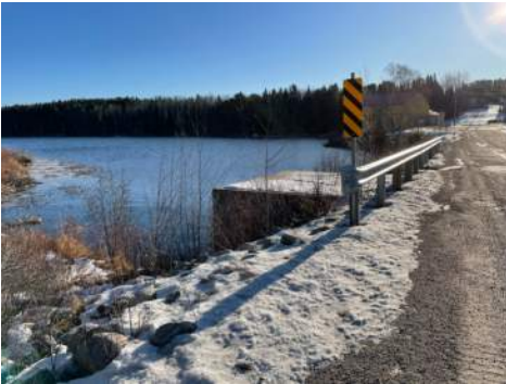
Downstream looking East
