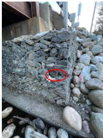
Slope Protection - SU2. Note: Typical holes in gabion wires.
