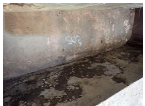
SU2 Abutment wall - between G1/G2. Note: Disintegration of bearing seat.
