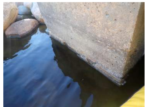
Outlet - SE corner. Note: Disintegration of concrete footing below waterline.
