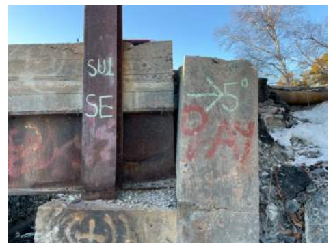
Foundation - SE. Note: Gap between decktop and ballast wall at SU1
