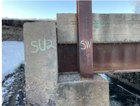
Foundation - SW. Note: Gap between deck top and ballast wall at SU2
