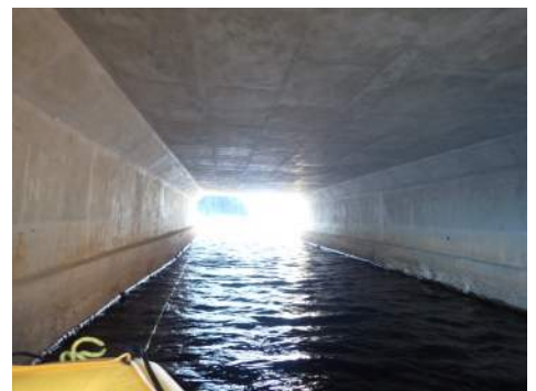
Looking towards inlet from outlet.
