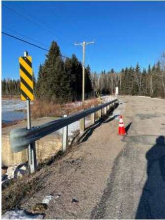
Typical West railing.
