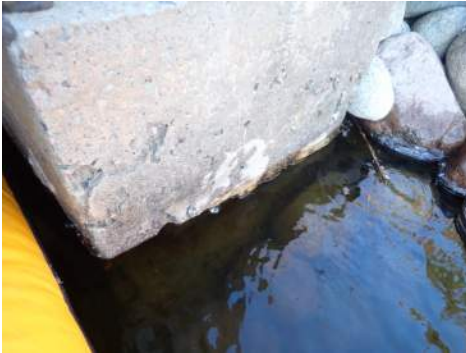
Outlet - NE corner. Note: Disintegration of concrete footing below waterline.
