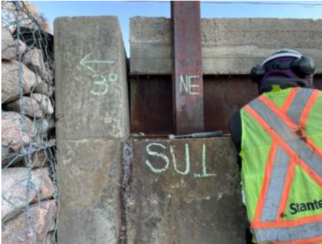
Foundation - NE. Note: Gap between deck top and ballast wall at SU1
