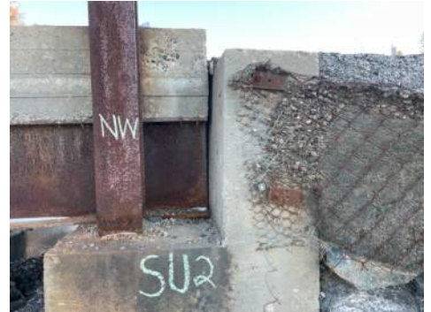
Foundation - NW. Note: Gap between deck top ballast wall at SU2
