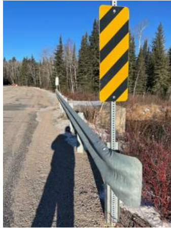
Typical East Railing
