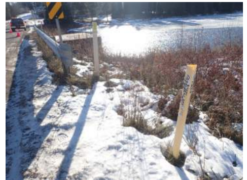
NW Embankment. Note: Utility markers.
