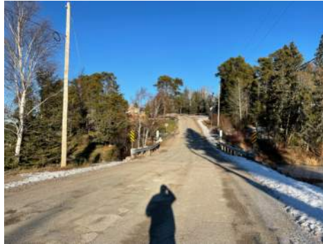
Roadway looking East
