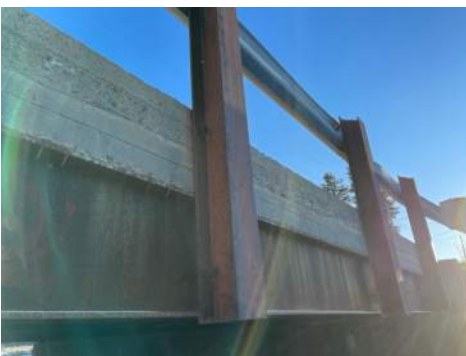
Typical North posts
