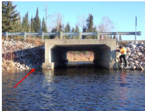
Embankments - West elevation. Note: Slight scour of NW embankment toe.
