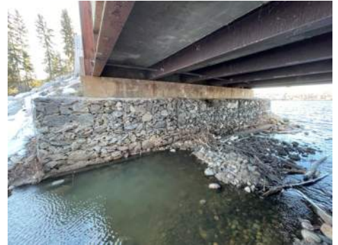
SU2 West abutment
