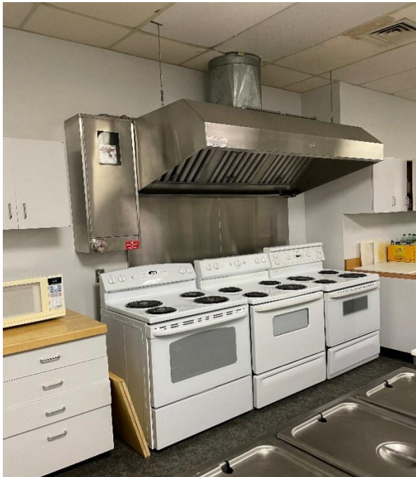
Figure 7– Community Hall's exhaust hood & fire suppression
