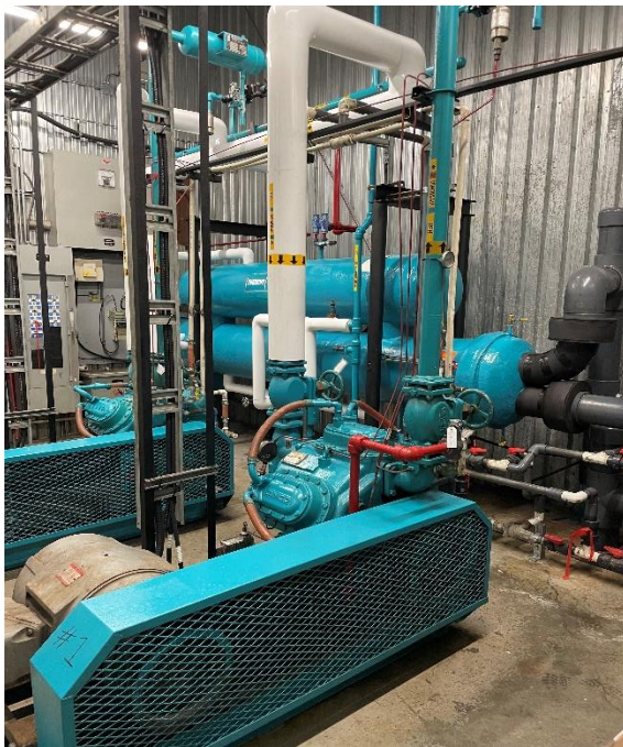
Figure 23– Ammonia refrigeration compressors and evaporator
