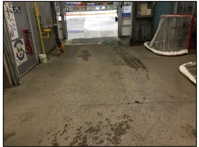
Figure 15 – Cracking and spalling of concrete slab in Ice Resurfacer Room
