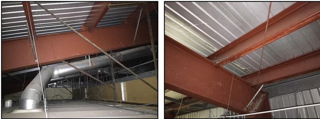
Figure 24 – Structural Steel Framing in the Community Hall
