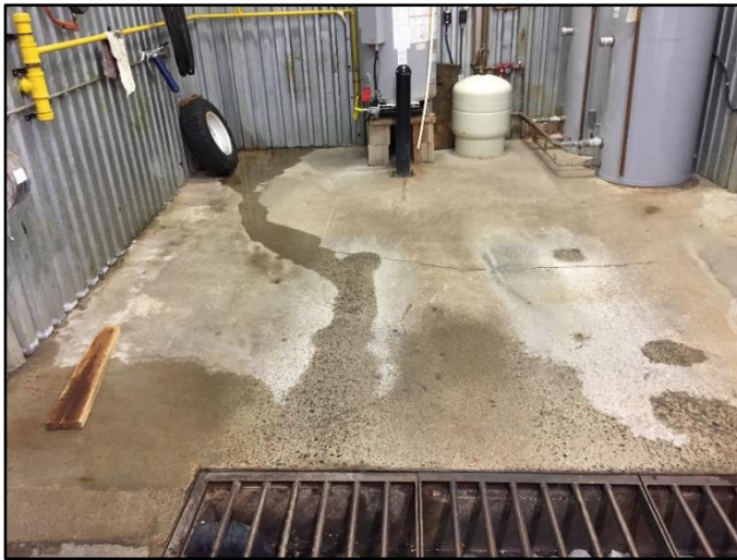
Figure 15 – Cracking and spalling of concrete slab in Ice Resurfacer Room
