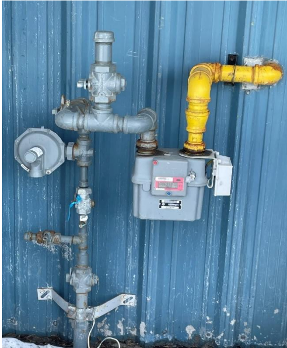
Figure 33– Natural gas service to ice rink water heater
