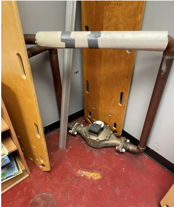
Figure 13 – Arena Hall's 2" domestic cold water supply
