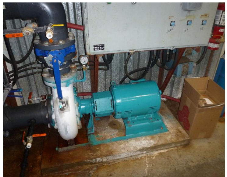
Figure 24– Frosted brine pump impeller casing
