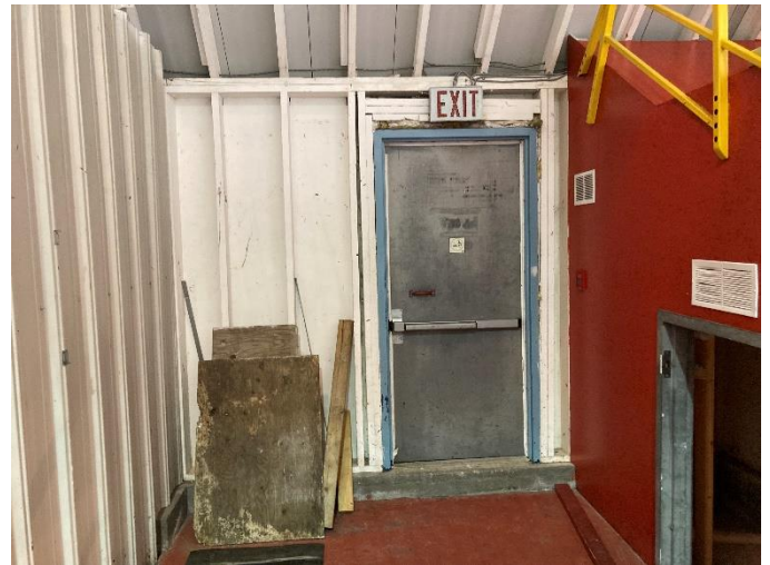
Figure 6 – Exit door with concrete curb from rink not meeting accessibility requirements
