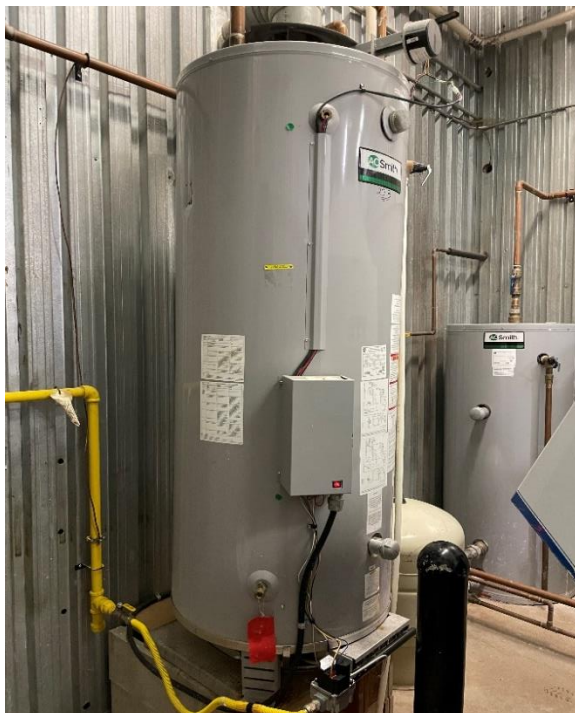
Figure 31– Ice rink gas-fired water heater
