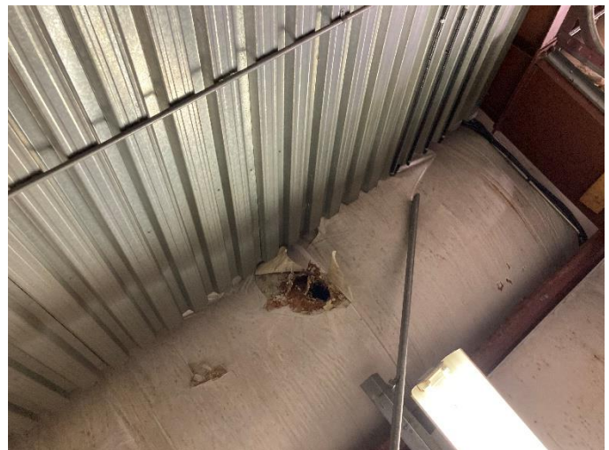
Figure 8 – leaks and damage to roof in ice resurfacer room
