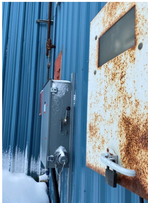
Figure 2 – Meter and portable generator plug-in
