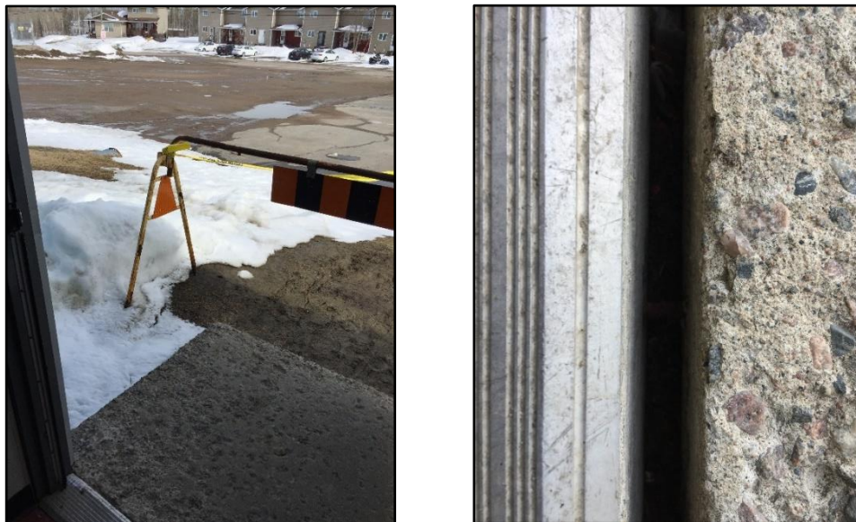
Figure 20 – Exterior concrete pad deteriorations near dressing rooms area
