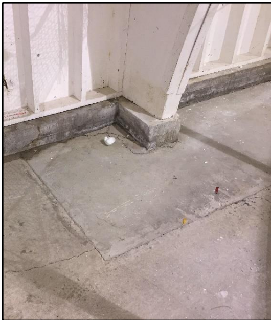
Figure 8 – Cracks in concrete slab near pilaster
