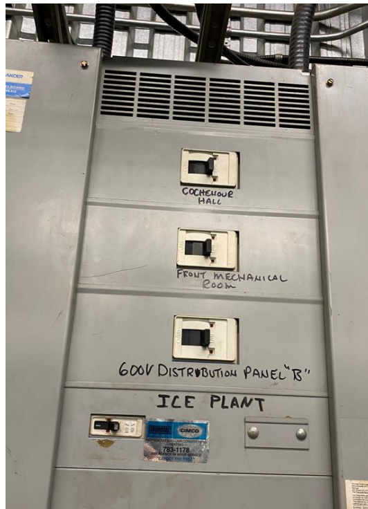
Figure 4 – Main Distribution Panel
