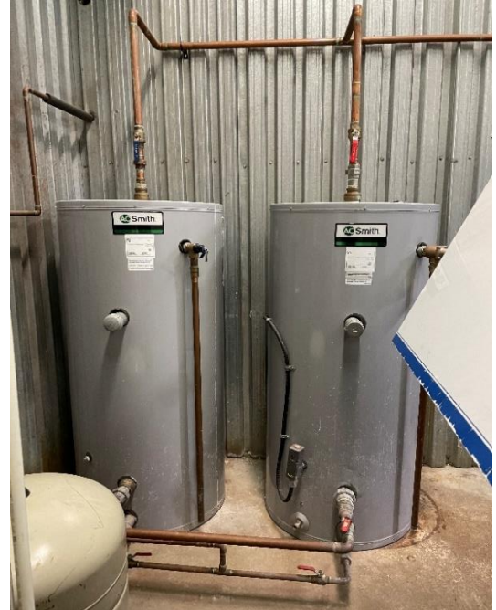
Figure 30– Ice rink electric water heaters
