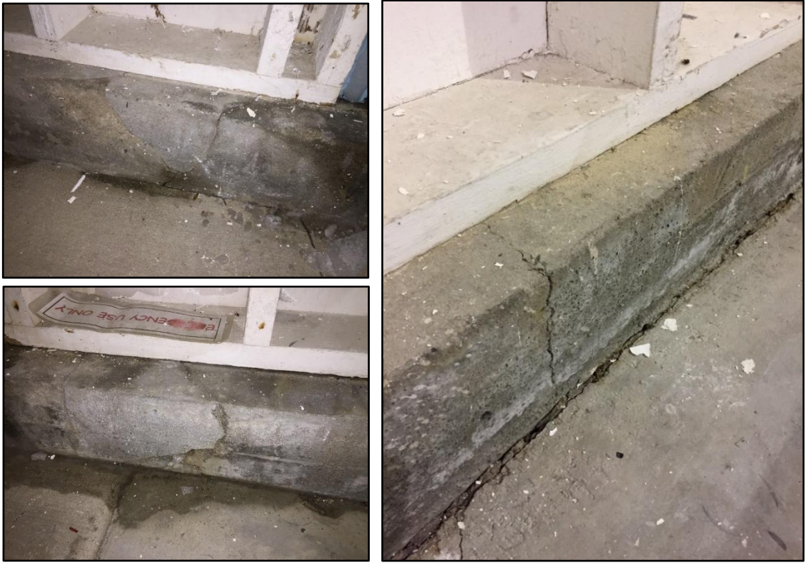
Figure 10 – Crack in grade beam at the north-west corner of the arena
