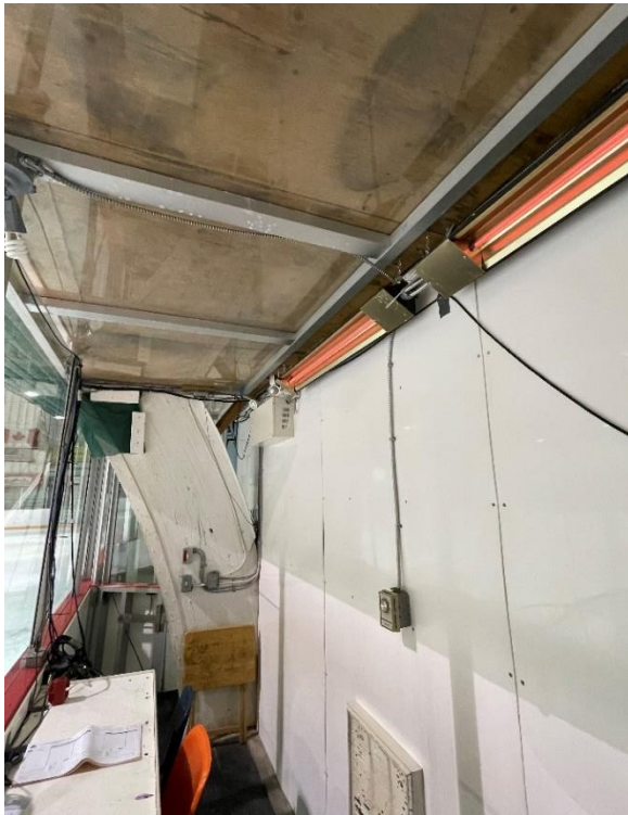
Figure 21– Scorer's electric infrared radiant heaters
