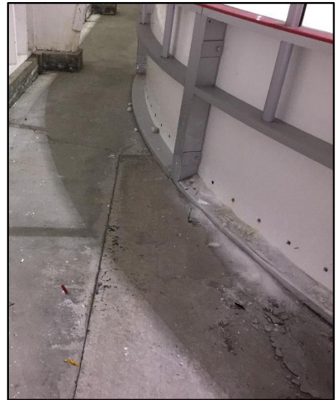
Figure 7 – Concrete floor cracks under ice board to the north-west corner of ice rink
