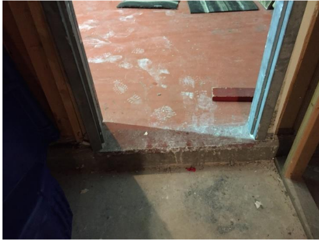
Figure 12 – Difference in concrete slab elevation
