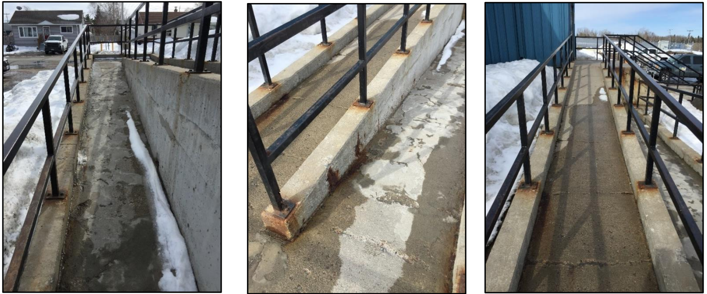
Figure 19 – Concrete ramp deterioration in front of the reception area
