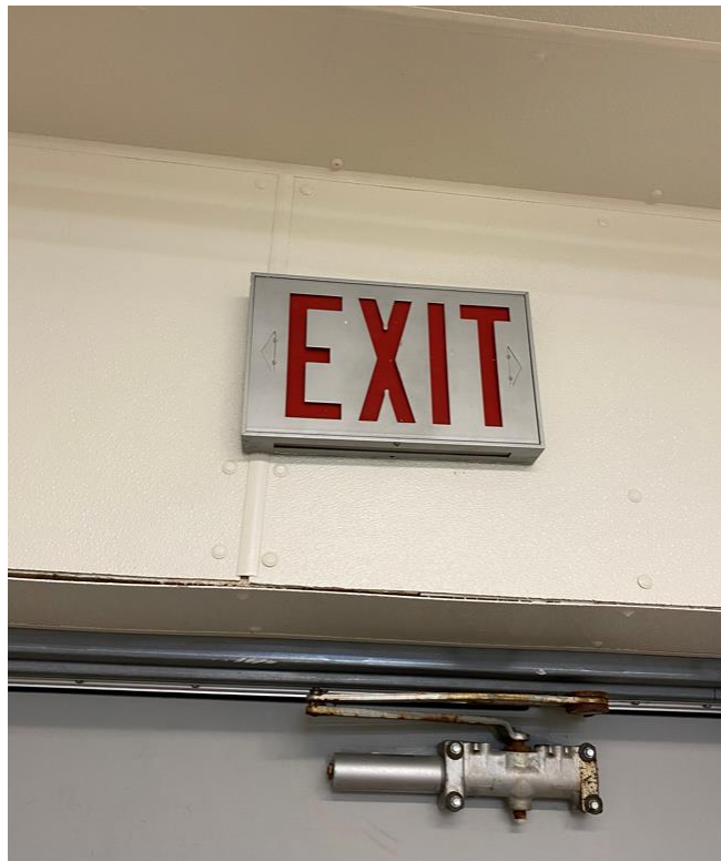
Figure 21 – Exit sign (no longer functional)
