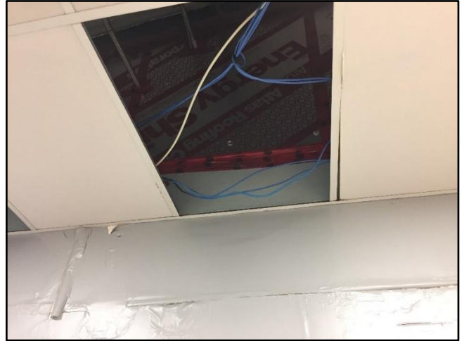
Figure 13 – Insulation at the wall between Hockey Arena and Reception Area
