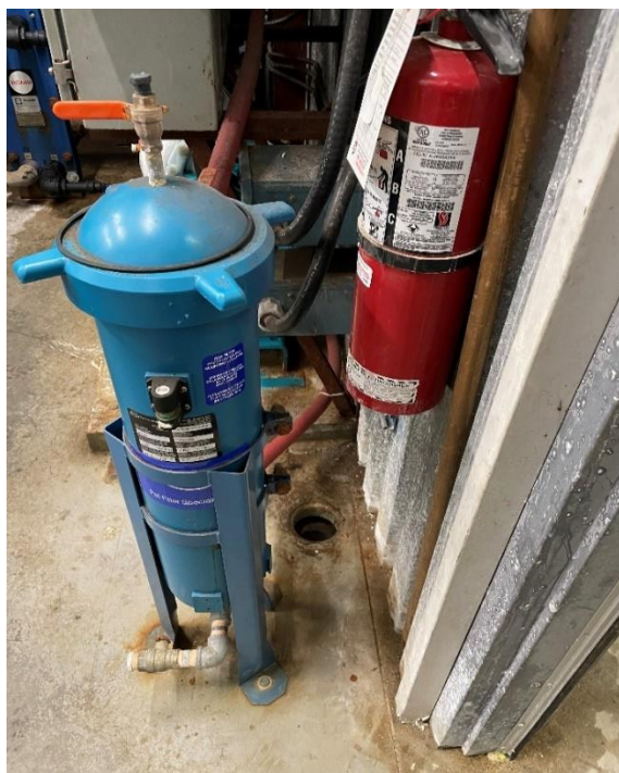
Figure 27– Filter unit and floor drain
