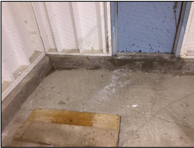
Figure 6 – Cracks in grade beams and concrete
