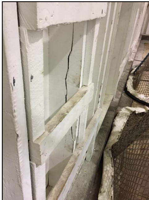
Figure 3 – Cracked stud at west wall of the arena.
