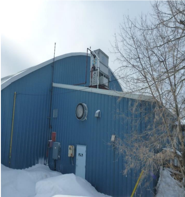
Figure 29– Cooling tower and wall-mounted centrifugal exhaust fan
