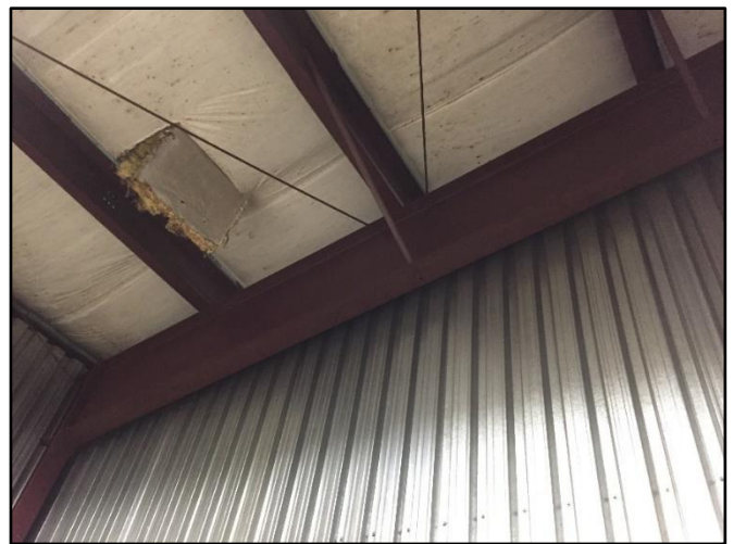
Figure 14 – Damage in Ice Resurfacer room roofing membrane
