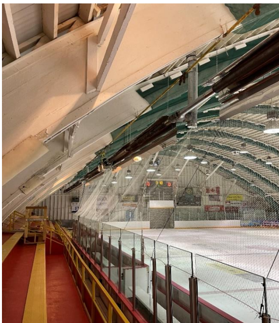
Figure 19– Seating/bleacher's radiant tube heaters
