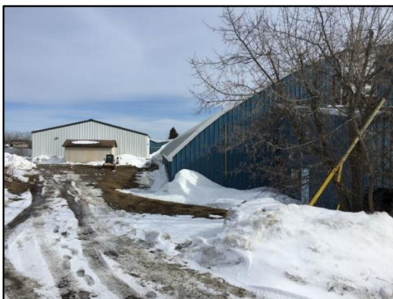
Figure 28 – Ground slopes towards north wall of the arena room slab.
