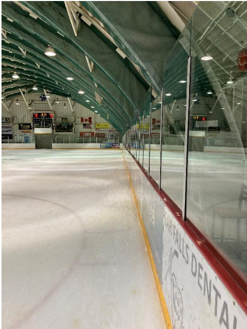
Figure 9 – glulam structure interfering with dasher board glass
