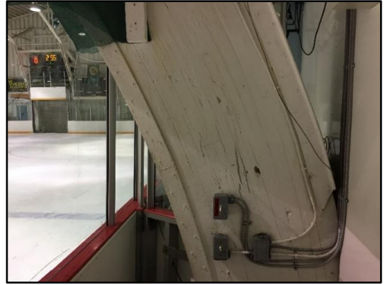
Figure 2 – Cracks in the glulam arched beams indicating delamination.
