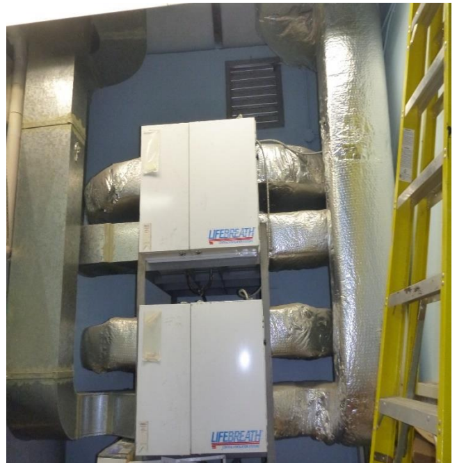
Figure 16– Arena dressing room ventilation units
