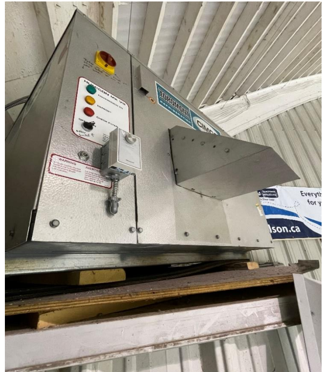
Figure 22– Ice Rink's dehumidifier
