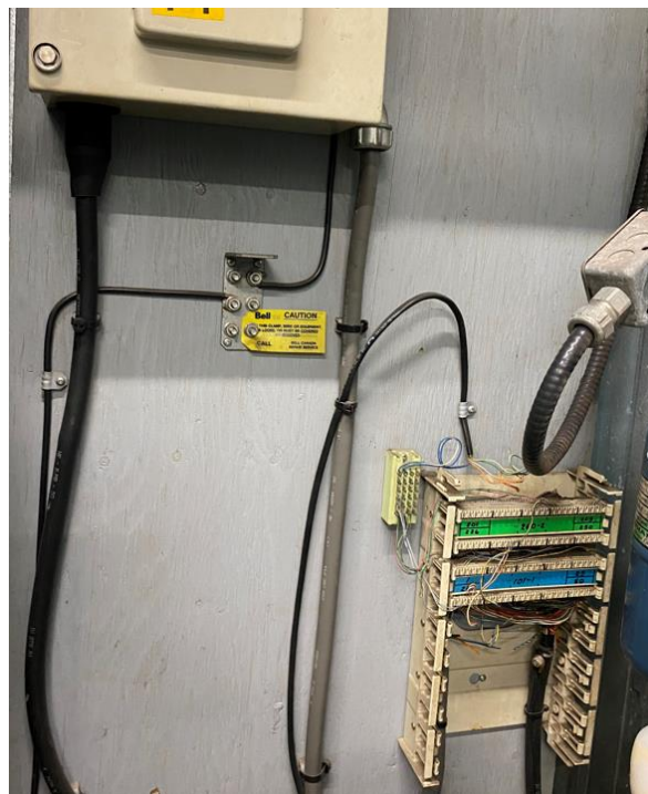
Figure 16 – Tbaytel termination in the [back] mechanical room
