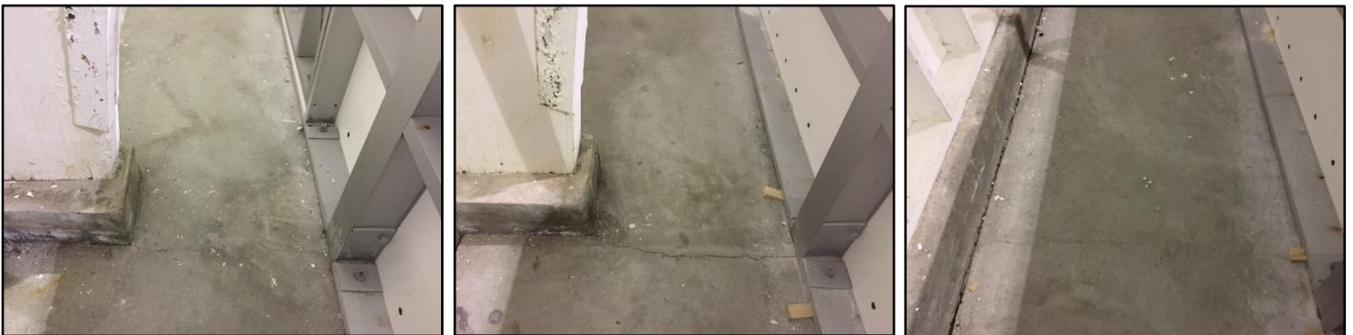
Figure 11 – Slab-on-grade shrinkage cracking
