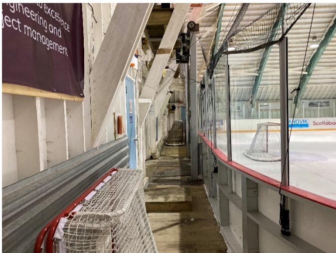
Figure 7 – cover over header trench for chilled slab and access to ice plant
