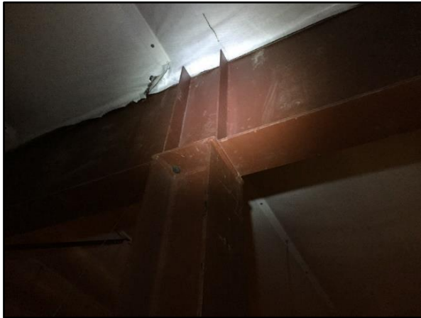
Figure 17 – Structural Steel Framing in the Reception Area
