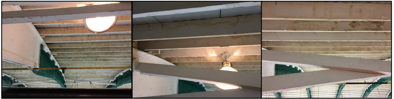
Figure 4 – Wood purlins in the arena
