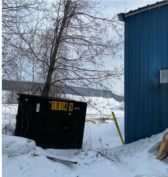
Figure 1 – Utility transformer
